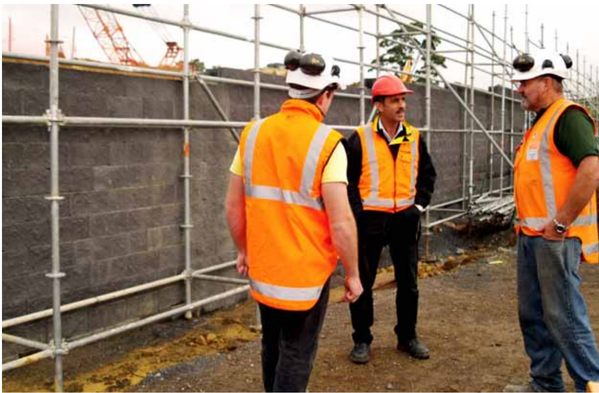
Namir Asmaro (centre) with the Site Engineer and Site Foreman from Fletcher Construction
