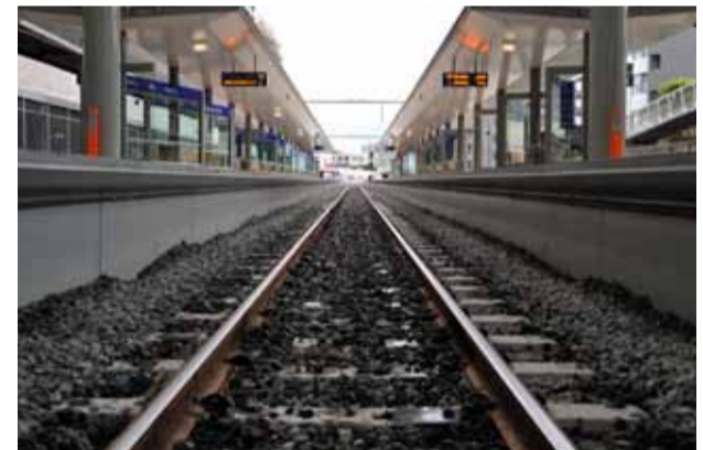
Ballast at Newmarket Station
