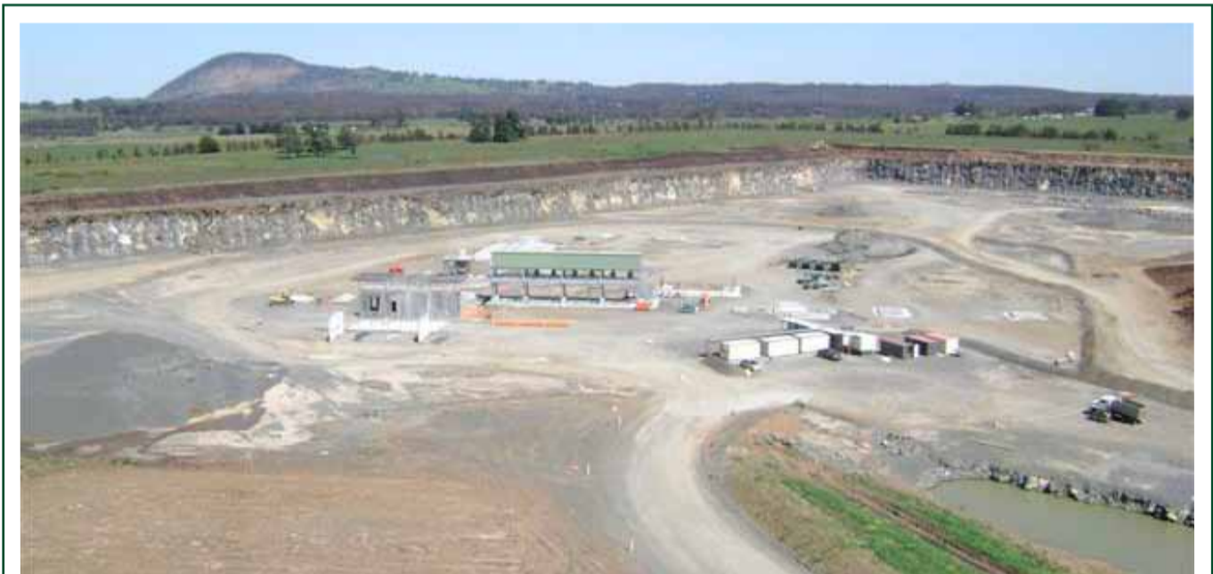
Boral Dunnstown reclaim tunnel and binset structure
