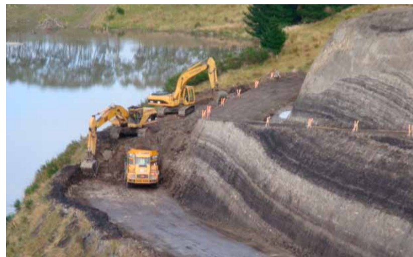
Rehabilitation work underway at Ohai mine
